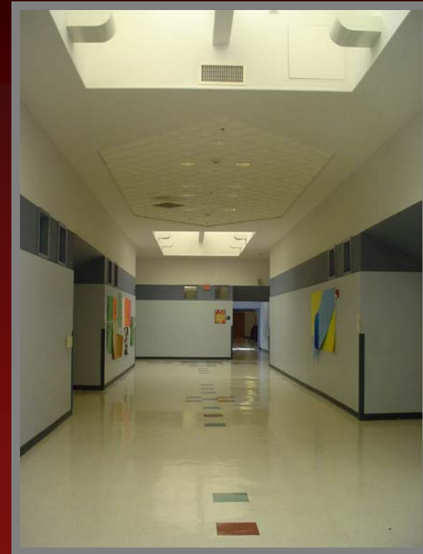
Maryvale Mall – skylights were utilized to compensate for a lack of windows in the boxy external structure
