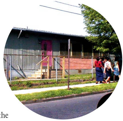
Temporary classrooms behind an East Orange high school relieve overcrowding but use up scarce open space.
